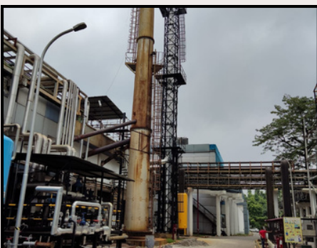
DG & BOILER CHIMNEY INSTALLATION & DISMANTLING
