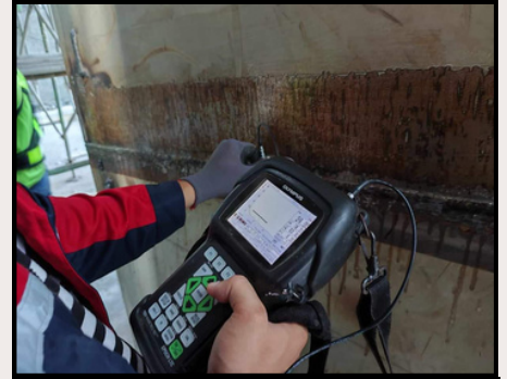
ULTRASONIC THICKNESS TESTING
