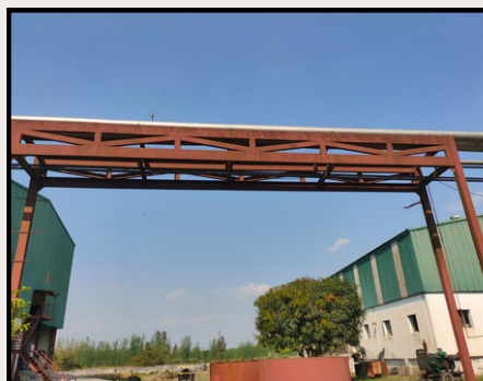
BRIDGE, STAIR PLATFORM FABRICATION
