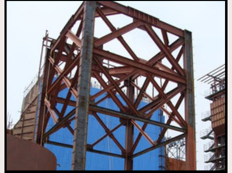
PLANT STRUCTURE FABRICATION
