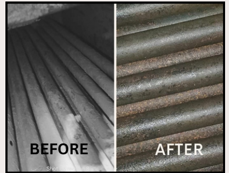
BOILER CHEMICAL CLEANING (DESCALING)
