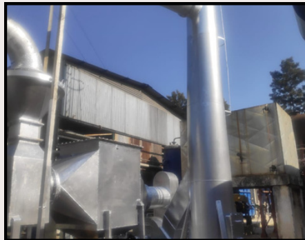
CHIMNEY & STRUCTURE PAINTING WORK
