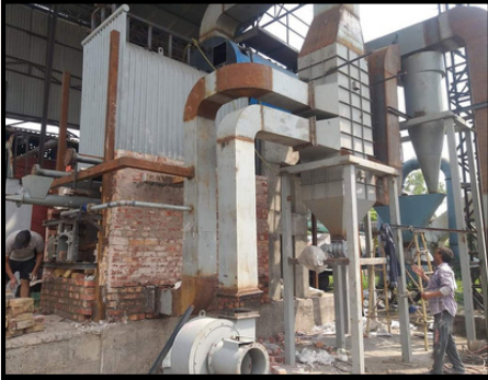
BOILER ERECTION SERVICE
