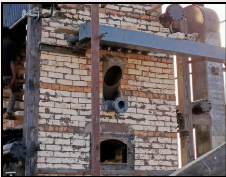
FURNACE REFRACTORY WORK
