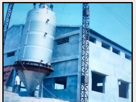
TANK, VESSEL LIFTING & SHIFTING
